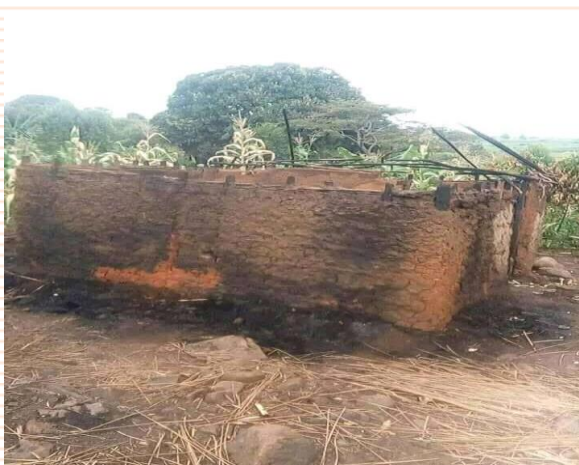
Burnt down house
